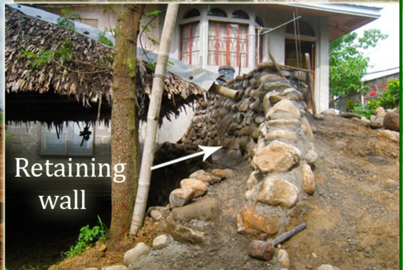
Grading property for our house
