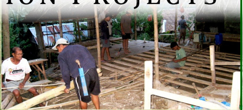
New addition to the church
